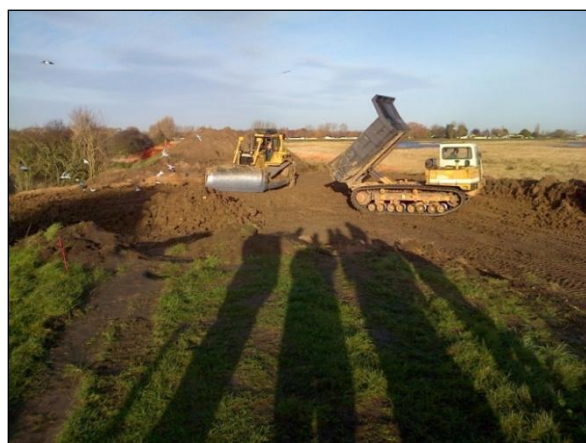
Tetney Marsh breach repairs – 20.12.13
