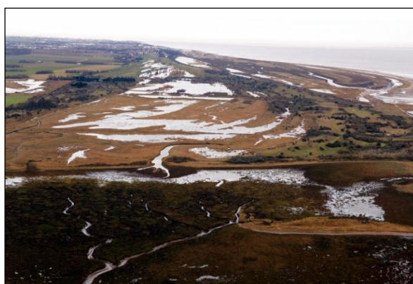
Bulldog Bank breach – Photo Taken by C J Helicopters
