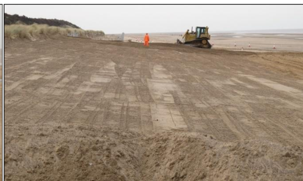
Mablethorpe emergency works
