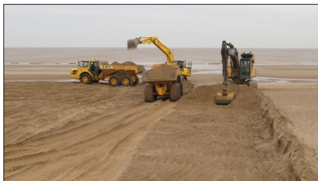
Mablethorpe emergency works
